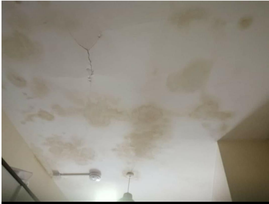
Figure 9 – Ceiling damp, House 16, 2021-22
