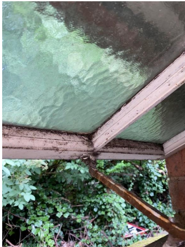
Figure 6 – Window mould, House 14, 2022-23
