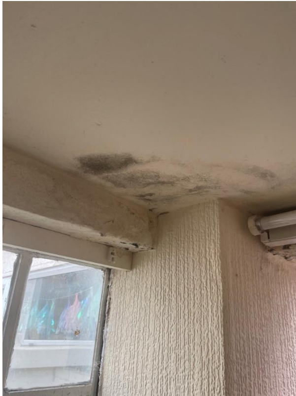
Figure 3 – Ceiling damp, House 5, 2022-23
