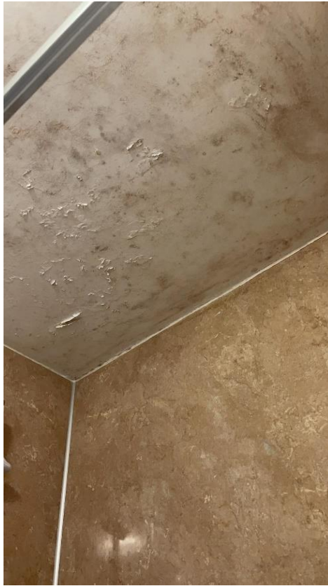
Figure 5 – Bathroom damp, House 9, 2021-22
